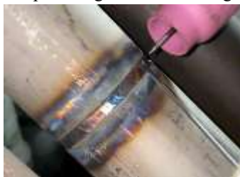
(a) Weld seam of kerosene pipeline
